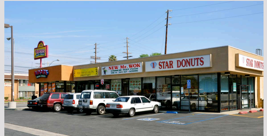
Subject Property, Northerly Building
