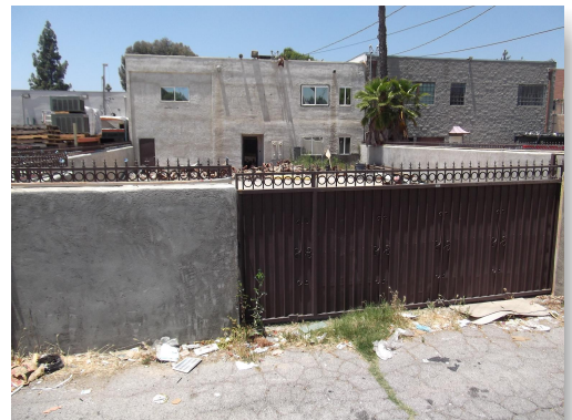
Rear building Parking space view
