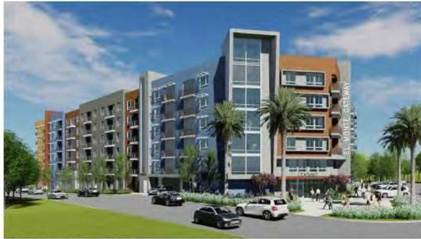
1. VIEW LOOKING NORTH-EAST
